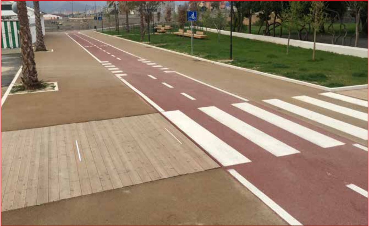
Savona: urban renovation of Zinola esplanade
