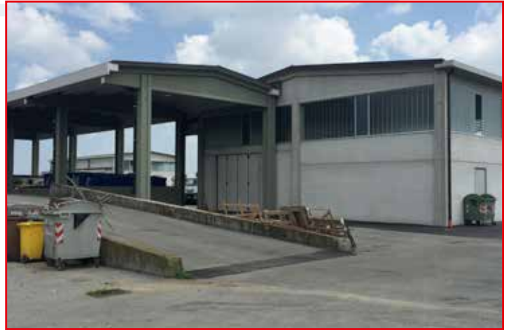
C.S.E.A. - Cuneo Ecology and Environment Services: demolition and rebuilding of the warehouse at the Revello collection platform
