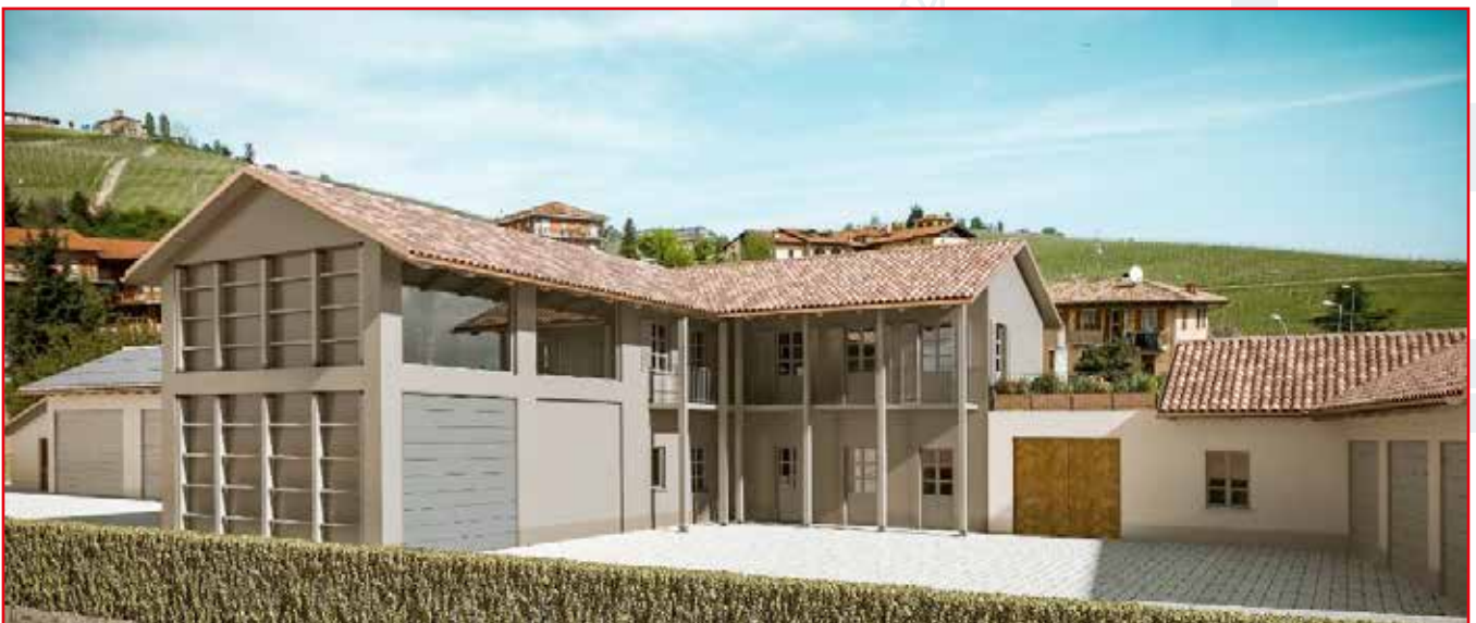
Barolo (CN): demolition and reconstruction of Mascarello wine producer cellar
